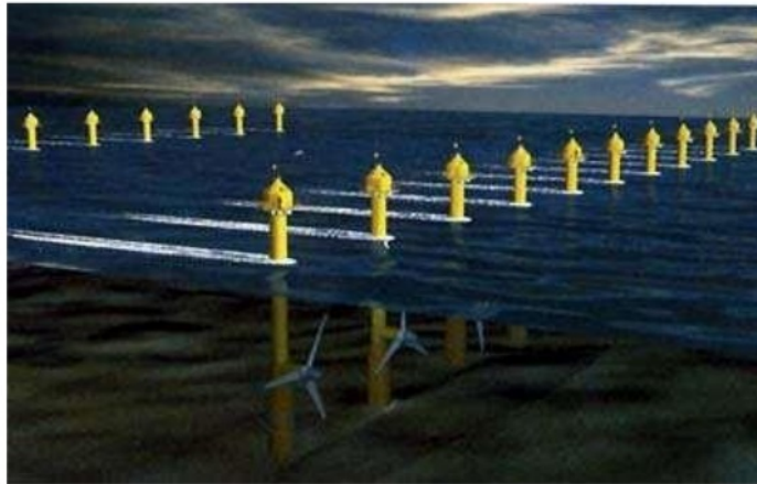
Fig.4 Installation of turbines on the seabed
